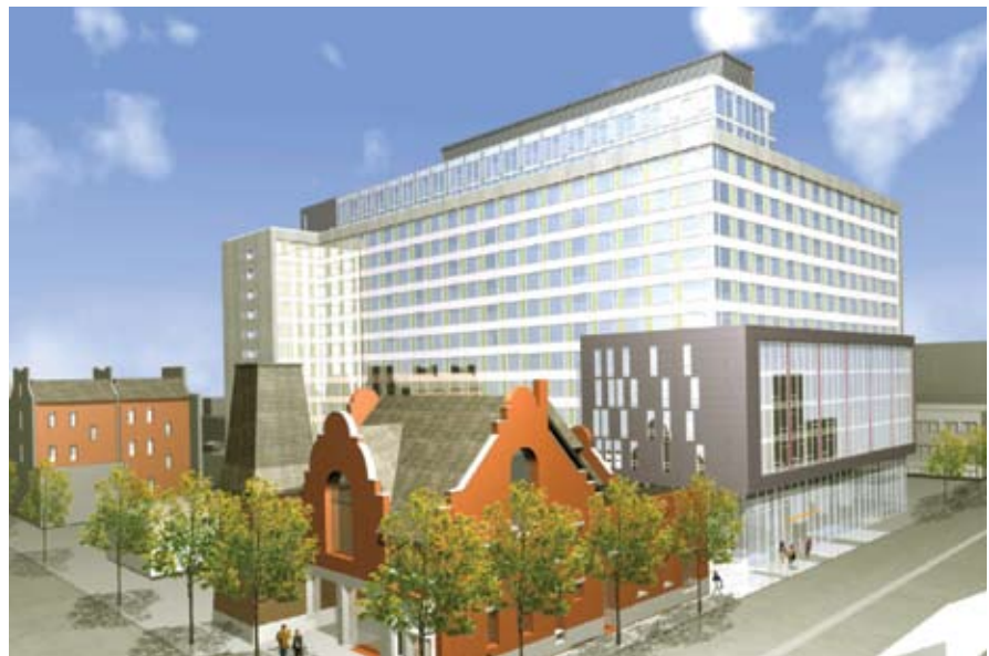
Toronto Community Housing's 501 Adelaide Street East, affordable rental for families to be complete in early 2009, features state-of-the-art environmental technologies.
